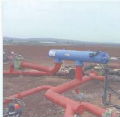
▲ Filtration of reservoir for drip irrigation, 130µm, ISRAEL
