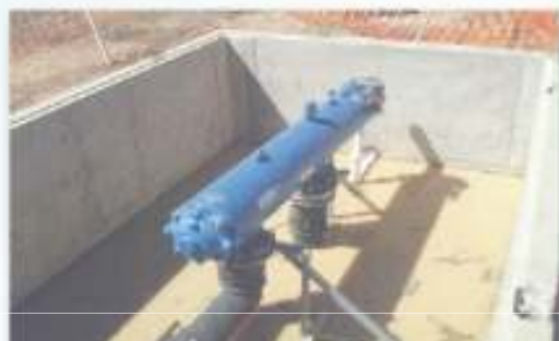
▲ Treated sewage effluent water for landscape irrigation, 130µm Sandhurst Estate, Carrum Downs(Melbourne), AUSTRALIA
