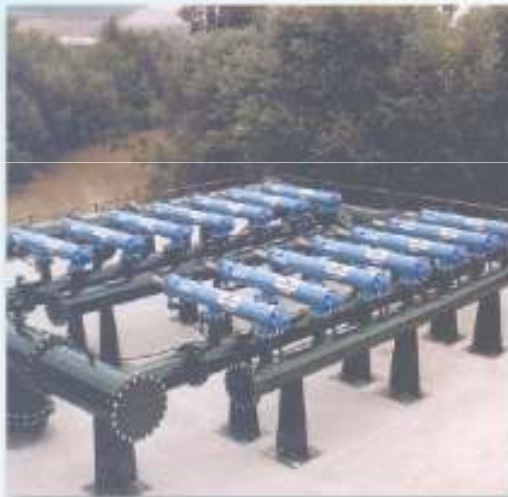
▲ River water filtration for drip irrigation, SPAIN
