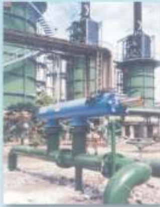
▲ Cooling water filtration at a power station, 100µm, CHINA
