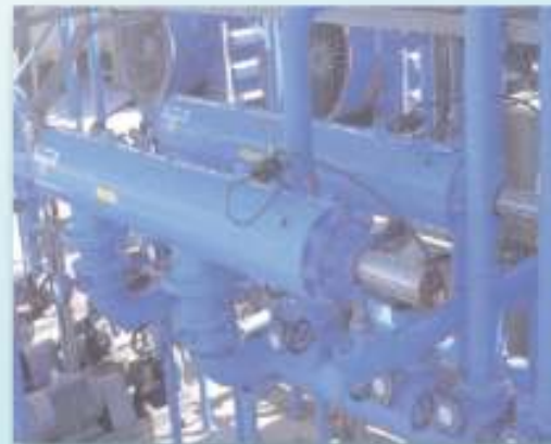
▲ Cooling water filtration, 50µm, Detergents manufacturer, ISRAEL
