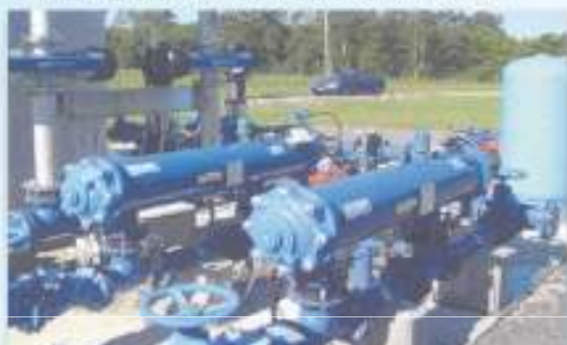
▲ Treated sewage water for irrigation of pasture, 200µm Stroud Sewage Treatment Plant, Stroud, NSW, AUSTRALIA
