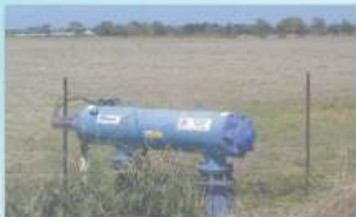
▲ Treated sewage effluent water for landscape irrigation, 200µm Bunnerong Cemetery, Bangholme(Melbourne), AUSTRALIA
